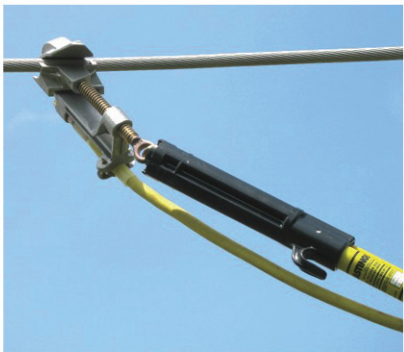
INSTALLING CLAMP
